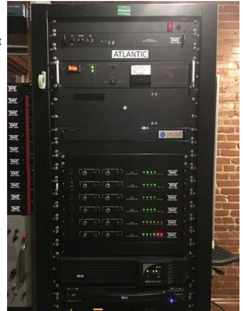
Rack mounted Ten Tec RX-331, one part of the receiver site in the systems still used for monitoring signals... Photo courtesy of Glen Pladsen AEØQ
