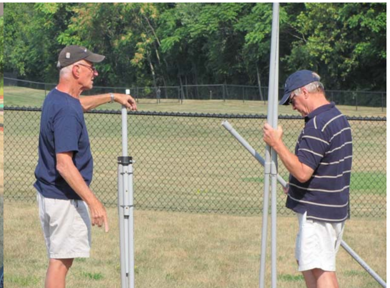
Below: K3VX & K3HCR assembling the 20 meter hamstick dipole support "structure" out of pre-cut PVC
