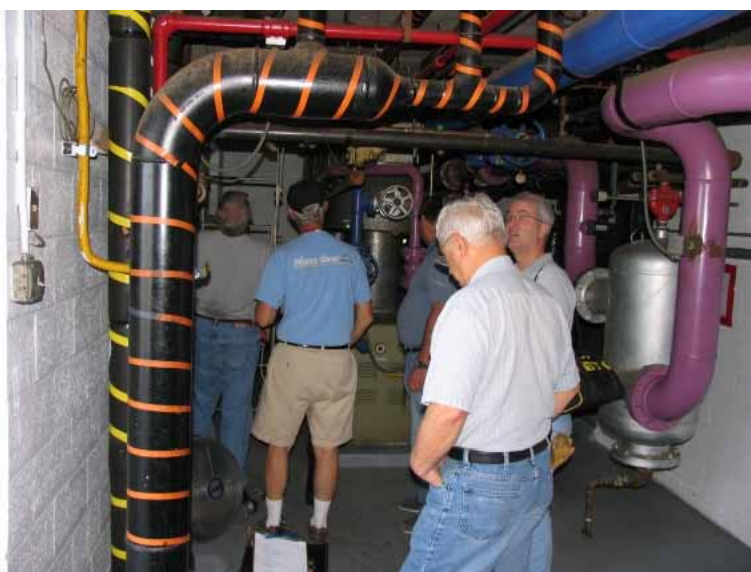
The mechanical room on top of the elevator shaft
