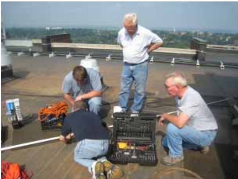
Above: Dismantling the repeater antenna
