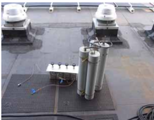
The duplexers see the light of day
