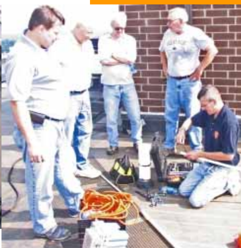
Working on the repeater antennas
