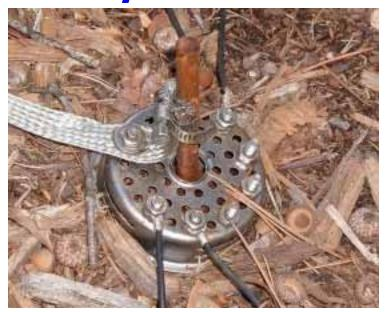
Depending on how many sets of stainless hardware you buy, the total cost for the strainer, the stainless steel screws, nuts and washers, and a small tube of Noalox will be under \$10 to maybe as much as \$16. For that price there's no excuse for not sprucing up (and adding to) your vertical's radial system.
