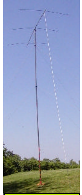
The 20 meter "Hamstick" Yagi, complete with Armstrong rotor (K3VX)
